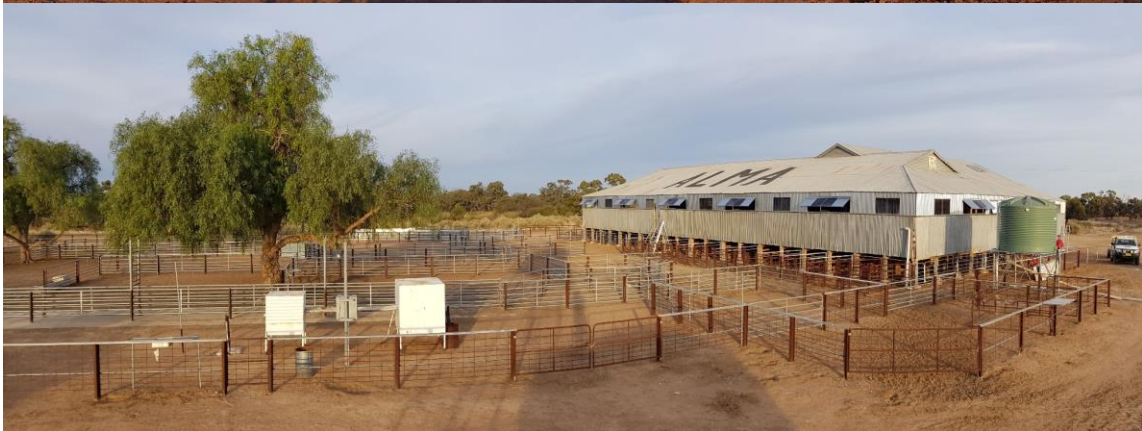
During (top) and after (bottom) woolshed renovations
