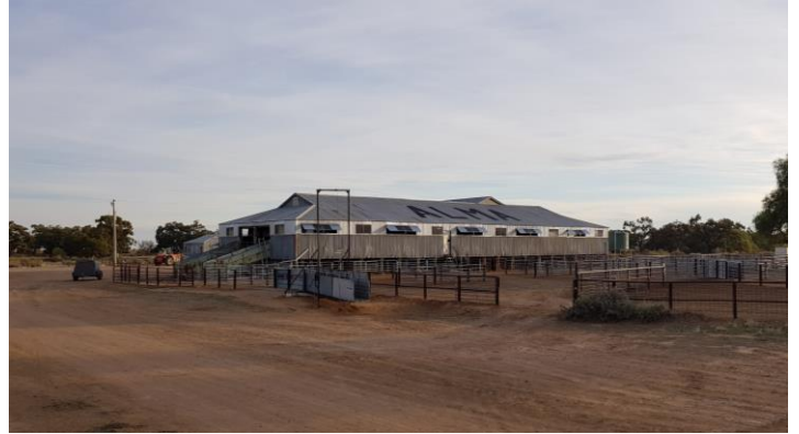
Alma woolshed with repaired foundations and new windows installed
